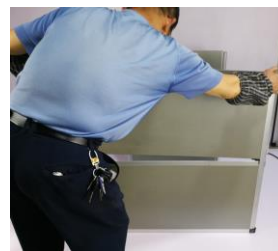
7: Insert the other bottom board into the alu connector.
